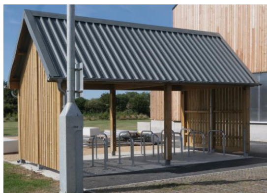
Convenient, overlooked, sheltered bicycle storage, the Arc, Chippenham
