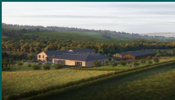
Hatchery at Preston Farm - Mcmullan Studio / Brick Visual
